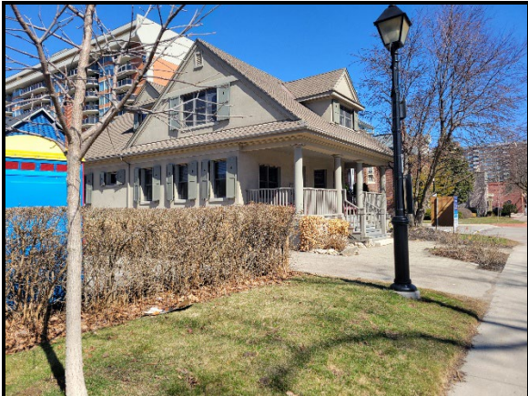
View of the abutting property to the east (1445 Ontario Street)
