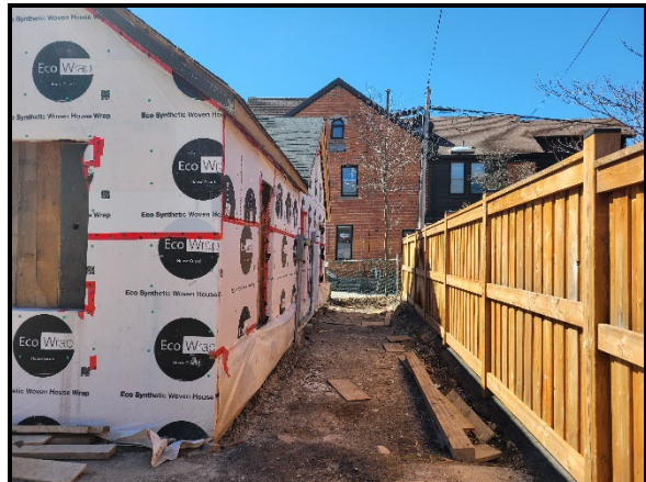
View of the rear of the property
