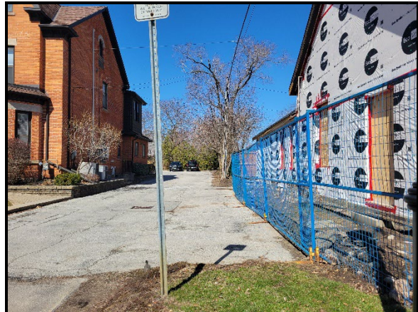
View of the westerly property line
