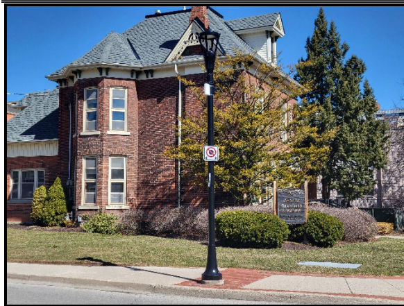
View of 1457 Ontario Street
