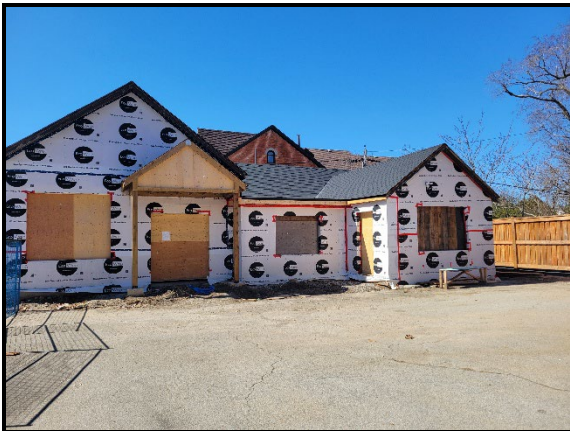
View of the east side from the parking lot
