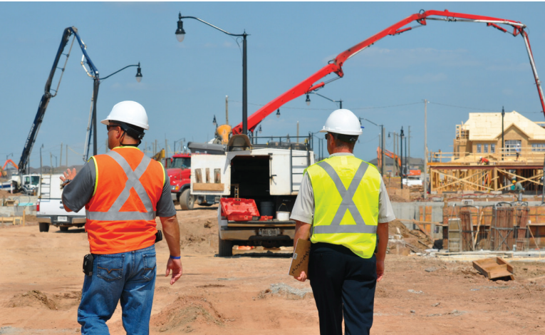
Employers and supervisors must ensure that their legal duties under the OHS and the requirements of the Construction Projects regulation (213/91) are met
