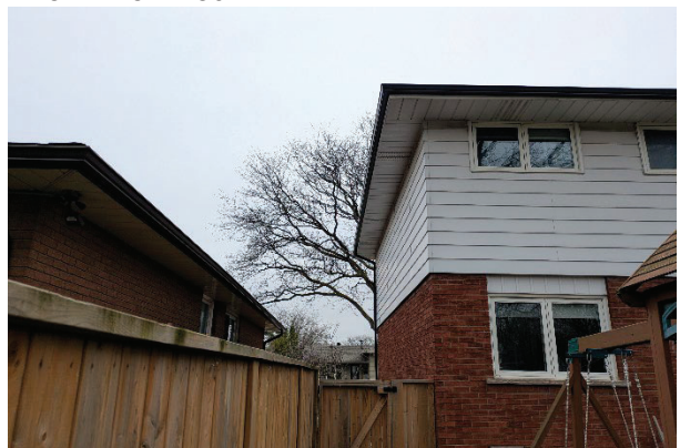
View of existing overhangs - from rear
