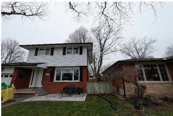
View of existing overhangs - from front
